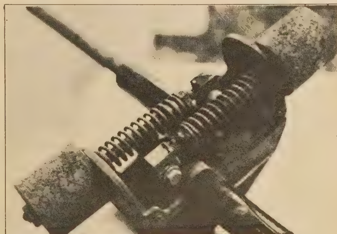
WINCHARGER GOVERNING DEVICES, ONE OF MANY THEY PRODUCED.
